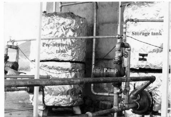
Fig. (12): Two storage tanks connected in series
