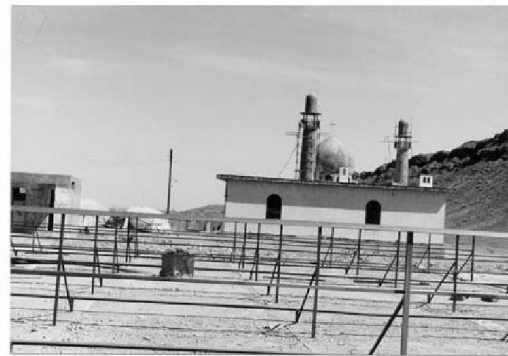
Fig. (8): The array support structure
